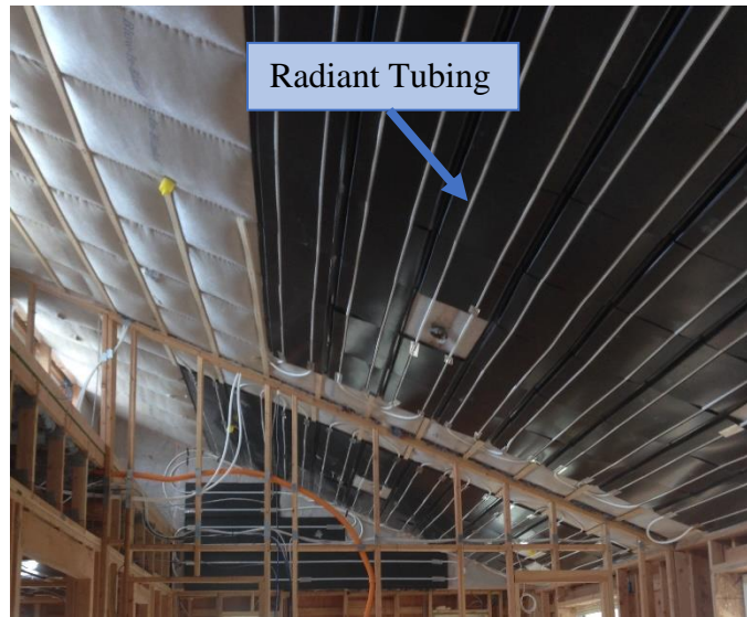
Figure 5. Installed radiant ceiling panels pre-drywall.
